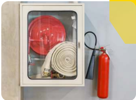
Hose Reel & Fire extinguisher
