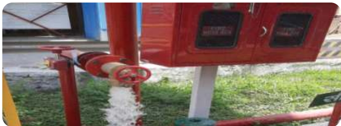
Fire hydrant Installation
