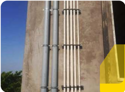
UPVC & CPVC Piping Installation
